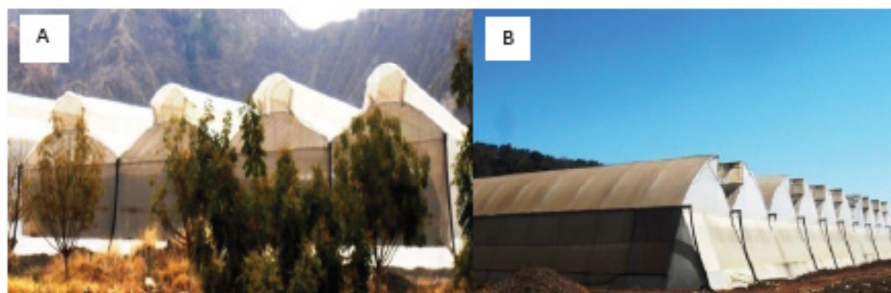
Figure 3. A. Multitunnel greenhouse type chapel in Jala, Nayarit. B. Multitunnel greenhouse type gothic in Tepic; Nayarit, Mexico. (Photography: L. Rodríguez R.).
